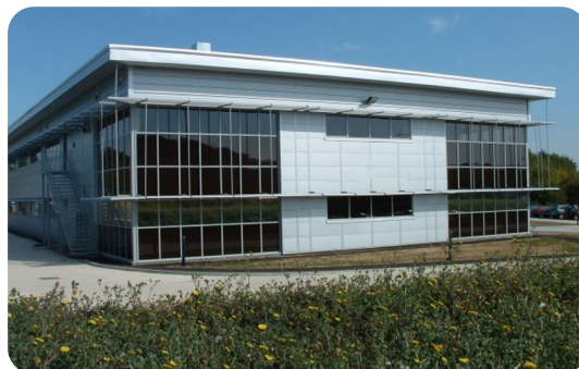
Haverhill, UK IVD Oligo Centre of Excellence
